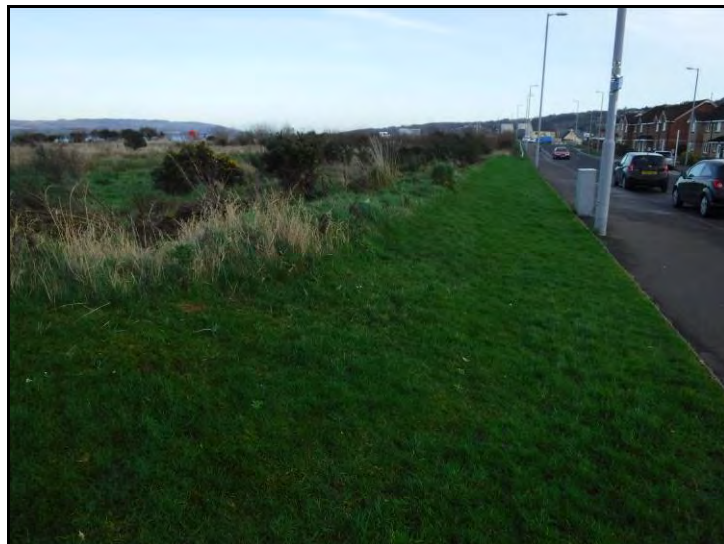
Plate 6 – View of the earthen embankment along southern edge
